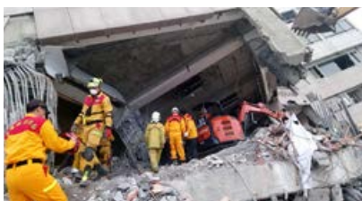
Collapsed building and relief activity by the firefighting department of Hualien Photo provided by the municipal government
