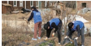
Removal of the vinyl cloth covering the soil
