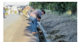
Cleaning up a ditch
